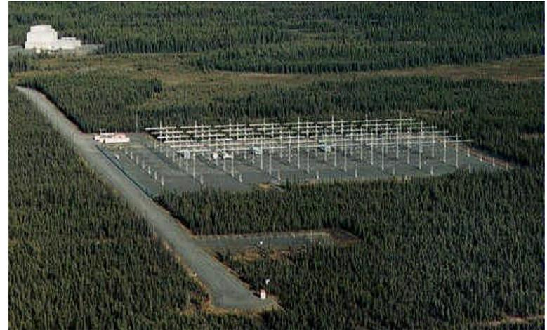
Above is an aerial view of the 48-antenna HAARP array. At top left is the Power Generation Building and Future Operations Center, to the left of the 48-Element HF Antenna Array is the Temporary Operations Center and the small structure at the bottom end of the runway is the Aircraft Alert Radar. The clearing above it is the Temporary Radiometer Pad.
